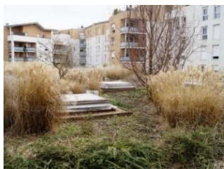
Toiture intensive (substrat 50 cm)
