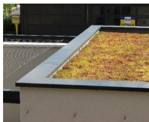
Toiture extensive (substrat 6cm)
